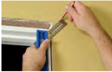
Lay Out Mitered Corners
